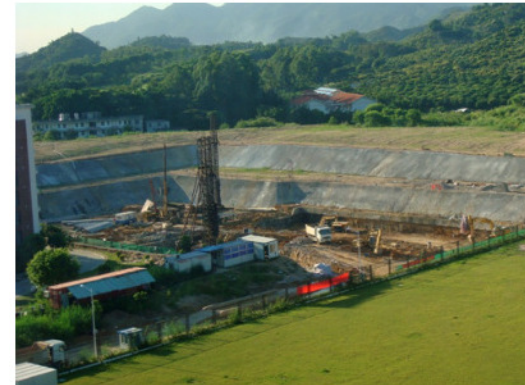
Under construction: China's massive new supercomputing center site in Shenzhen.
