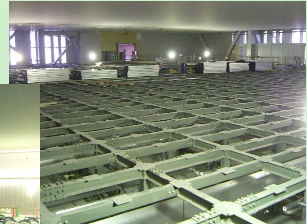
Making a double floor
